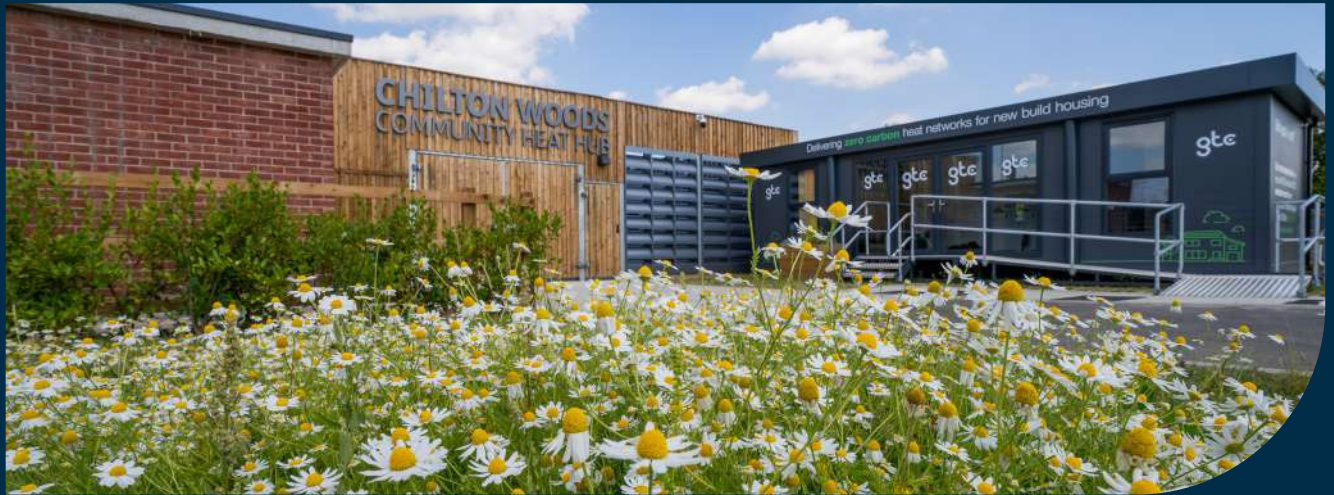
Chilton Woods Community Heat Hub.
