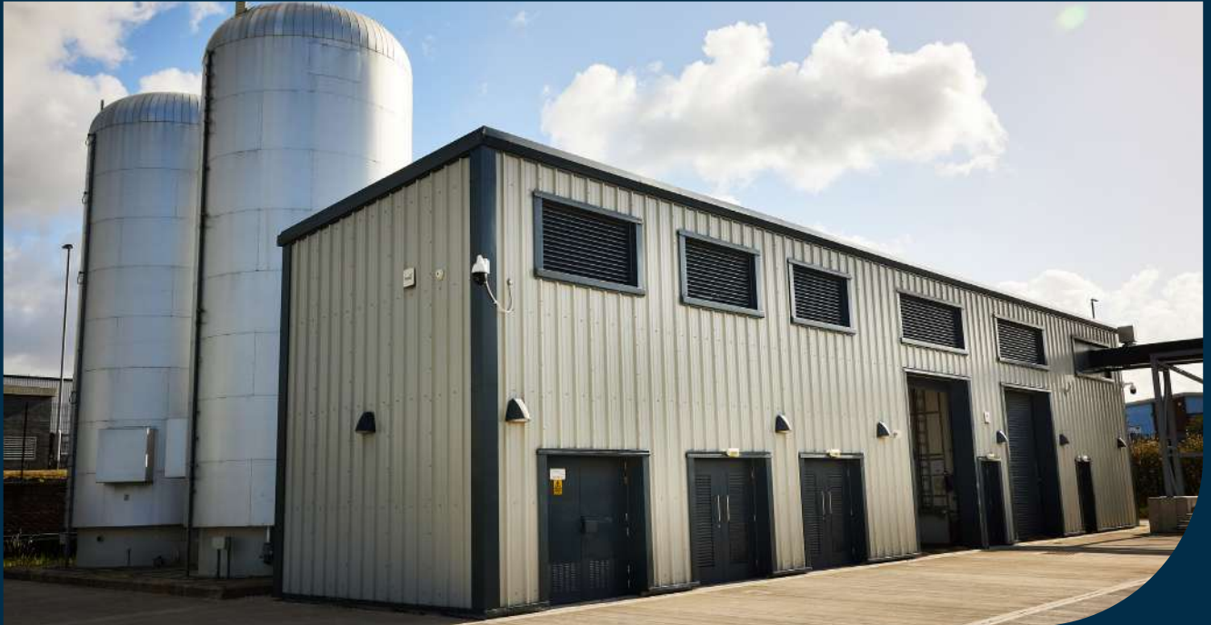
Energy Centre, Leeds. Courtesy of Vital Energi.
